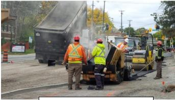
Placement of asphalt for cycle track
